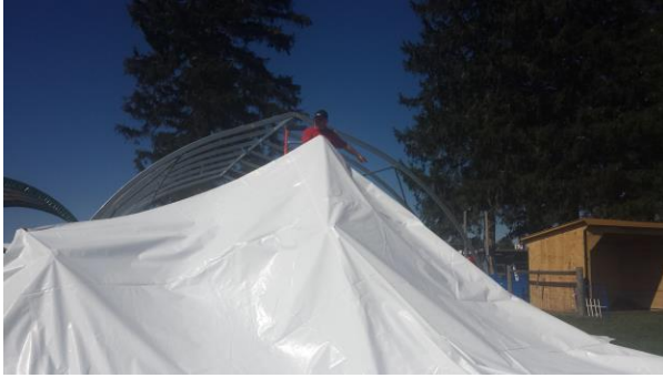
#43: pulling the cover over from the side, everyone takes a point of the cover to spread it out evenly
