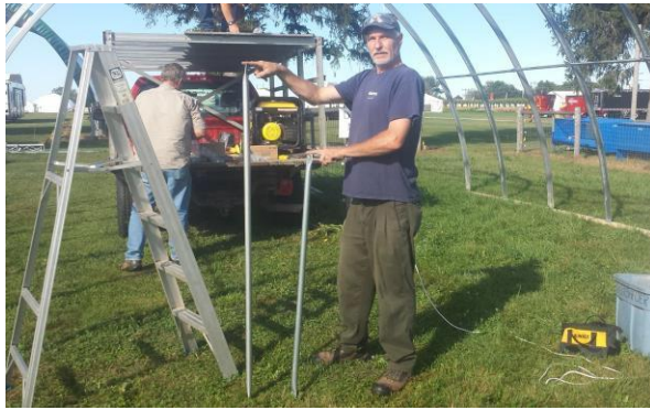
#19: IMPORTANT wind braces are the longer pipes, purlins are the shorter ones
