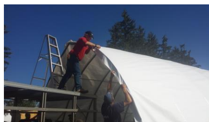
#54: keep the cover tight as you are working your way down with the wirelock
