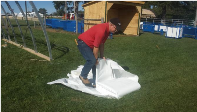
#37: lay out the covering
