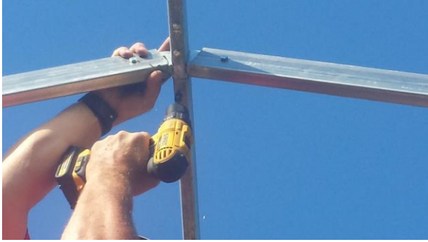
#18: secure the two sections of ridge together
