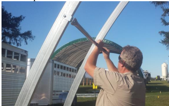
#19: IMPORTANT wind braces are the longer pipes, purlins are the shorter ones
