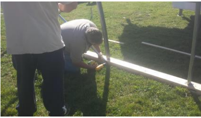
#30: complete wind brace Fastening
