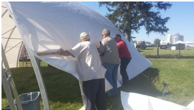
#56: ensure the screws are in the 1x2 to prepare for fastening the cover to the base
