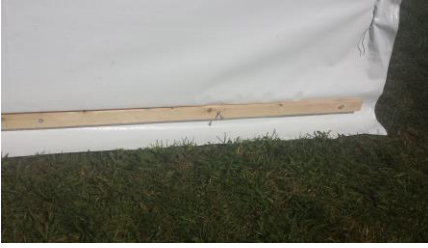
#62 & #63: completed cover fastening
