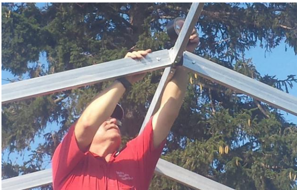
#17: wrap the joints of the ridge with duct tape
