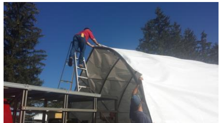
#49: pull to the end of the structure
