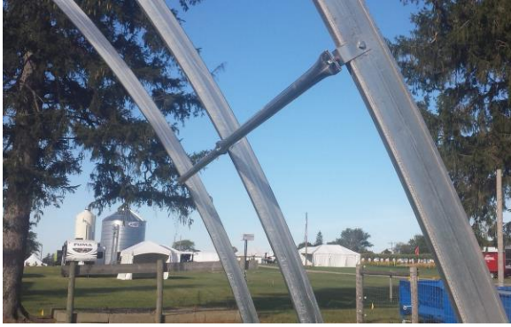
#21: purlins fastened with purlin clips to the hoop
