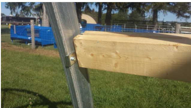
#35: attach the wood for roll up sides at the end hoop
