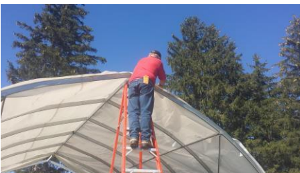
#53: put wirelock on both sides at the top
