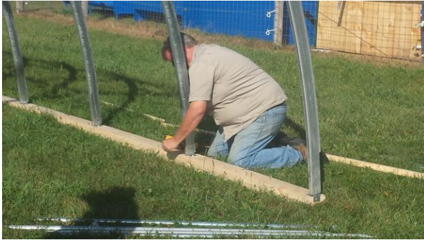
#33: put the #14 speed screw in the bottom of the hoop into the base bracket
