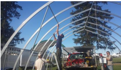
#26: secure the purlins along the line before completing wind brace fastening
