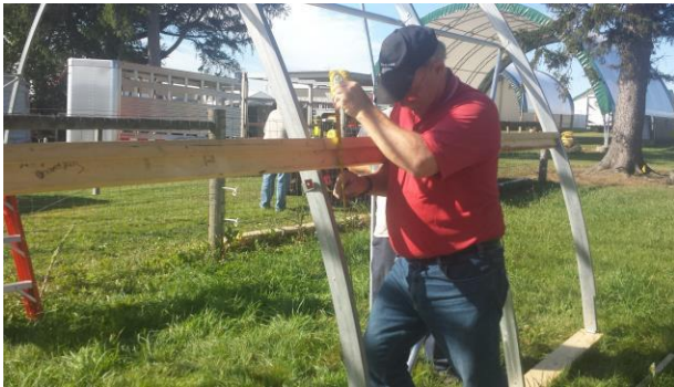
#34: measure for the roll up sides
