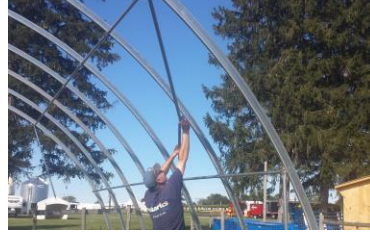
#29: complete wind brace fastening
