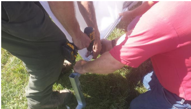
#65: fasten to the pipe, sandwiching the cover between
