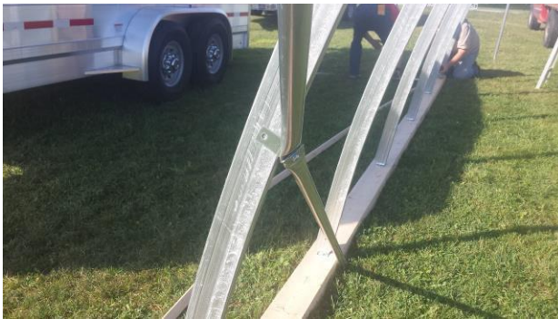
#32: completed wind brace fastening
