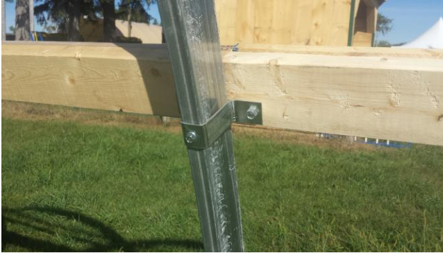
#36: attach the wood for roll up side
