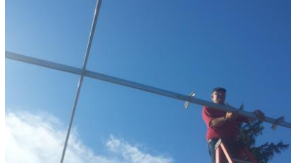
#15: connect the next section of ridge to the ridge starter at the end of the previous ridge section
