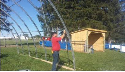
#28: tighten all fasteners to attach the wind braces
