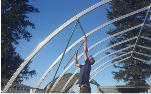
#25: secure the purlins along the line before completing wind brace fastening
