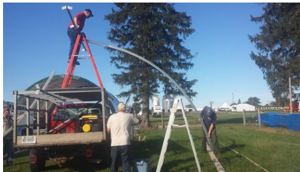
#4: flip the hoop right side up and slide it into the middle ridge stub
