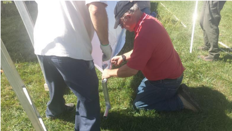
#64: roll the cover around the roll up pipe strap
