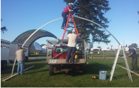
#5: get one pair of hoops standing attached to the middle ridge stubs before continuing
