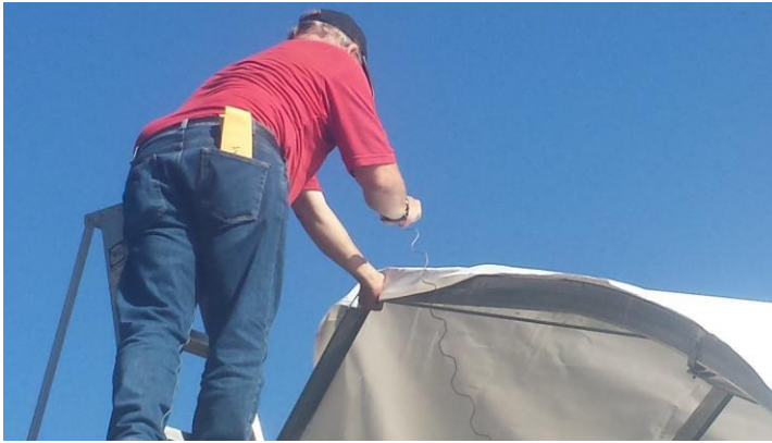
#50: pull tight and start wirelock at the ridge
