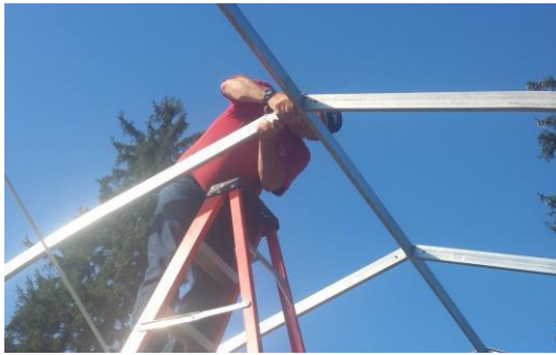
#16: make sure all hoops are fitting properly and secure
