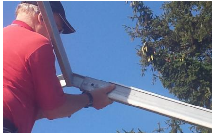
#7: slide the hoop into the ridge stub
