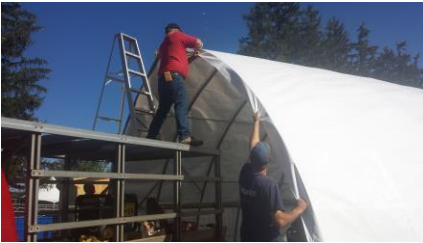
#51: pull the cover tight as the wirelock is going in
