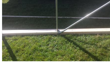
#31: wind brace lining up, not perfect, where it lands is good
