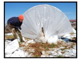
Take a 15' length of rope and tie the end hoop (top center) securely to one of the posts. Do this for both ends. This will prevent the hoop from being pulled laterally when you are tightening up the plastic later.
