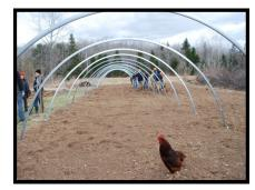
difficult to do later. If the ground is quite un even, it would be helpful to mark the rods for flat, or use a string line. Insert a safety clasp into the smaller hole of each base plate
